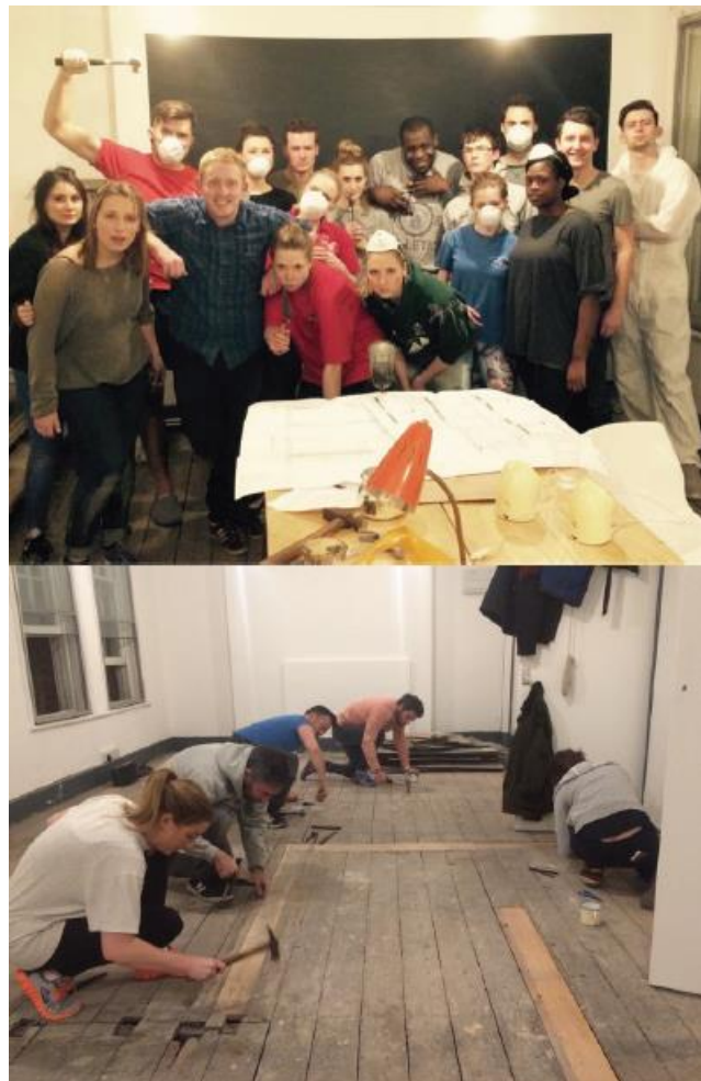
Members of the church volunteered to refurbish ARK
